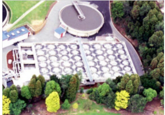
Energy efficiency is an important benefit of the aerobic FAST treatment system, installed at the Tokoroa Wastewater Treatment Plant.
