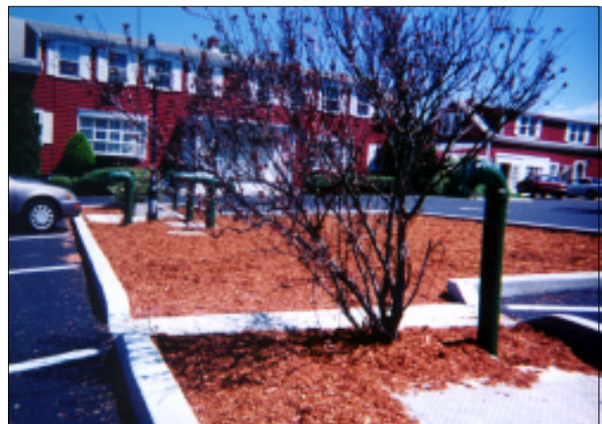
Smith & Loveless provided the Modular FAST® wastewater treatment system (top) to a historic hotel to help the facility maintain its seasonal variations of flow based on tourism. Placing the system underneath the parking lot (below), keeps the establishment aesthetically pleasing.
