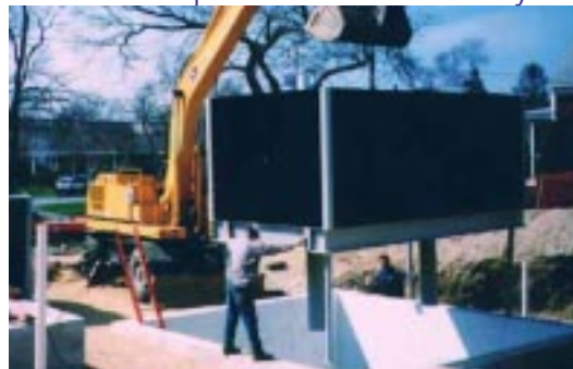
This system is easily installed into a small concrete basin.
