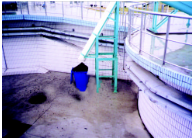
The result from a carefully considered grit handling, washing and dewater scheme is odor-free, dry grit for easy disposal.
